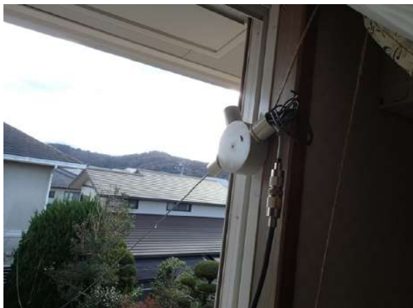
Fig. 6: Installation of the antenna
